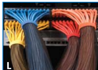
When cut with a hot knife, the sealed ends of PET allow for varied termination solutions.
